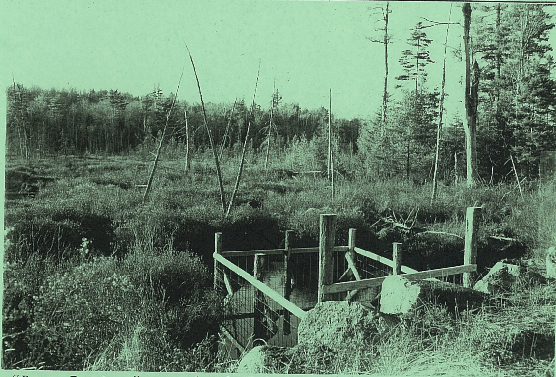
"Beaver Deceivers" are used on the Tribal Trust Lands to prevent road erosion and to protect the water quality of streams (Skip Lisle photo).
