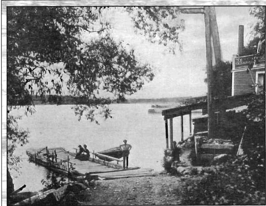
Orono to Bradley ferry landing
