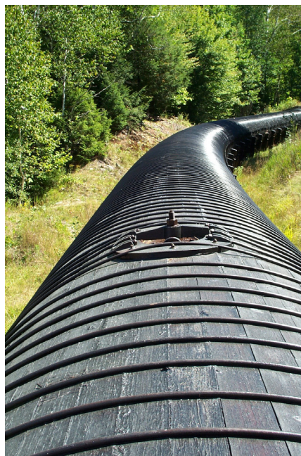
Somerset Reservoir Dam and outflow pipe in 2002.
